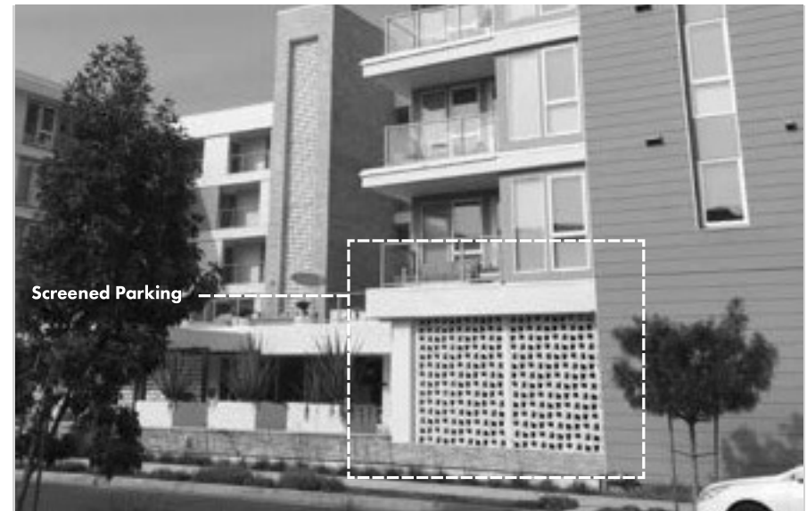
Figure 3.10: Example in an area of ground floor parking completely screened from view with decorative masonry ventilation blocks.
